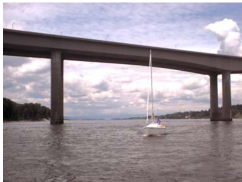
ISC's Cal 27" passes under the I-205 bridge
